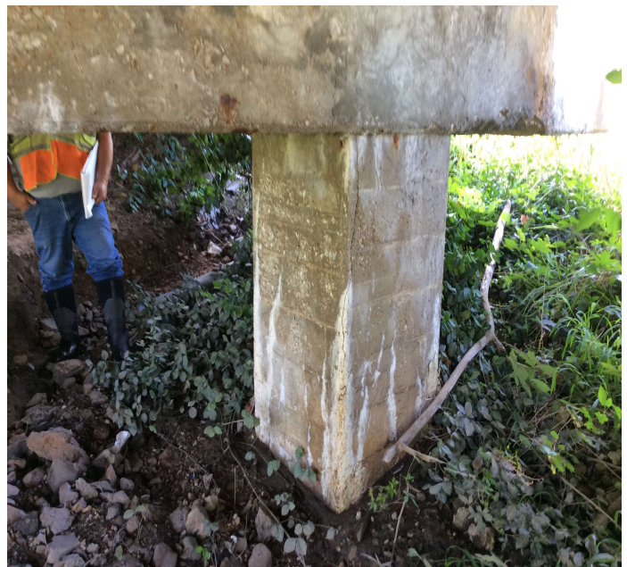
PHOTO 2 Description Efflorescent cracking to Right column @ Bent 3.
