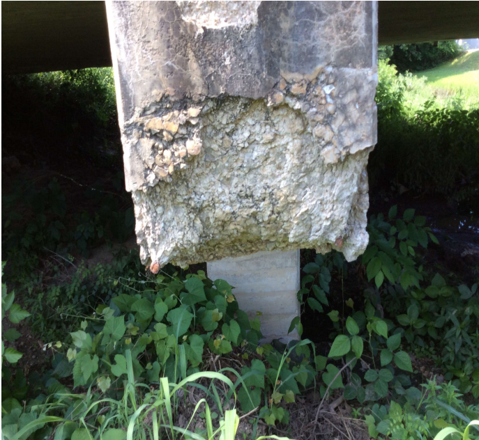
PHOTO 3 Description Deep spall to Left end of Cap @ Bent 3.
