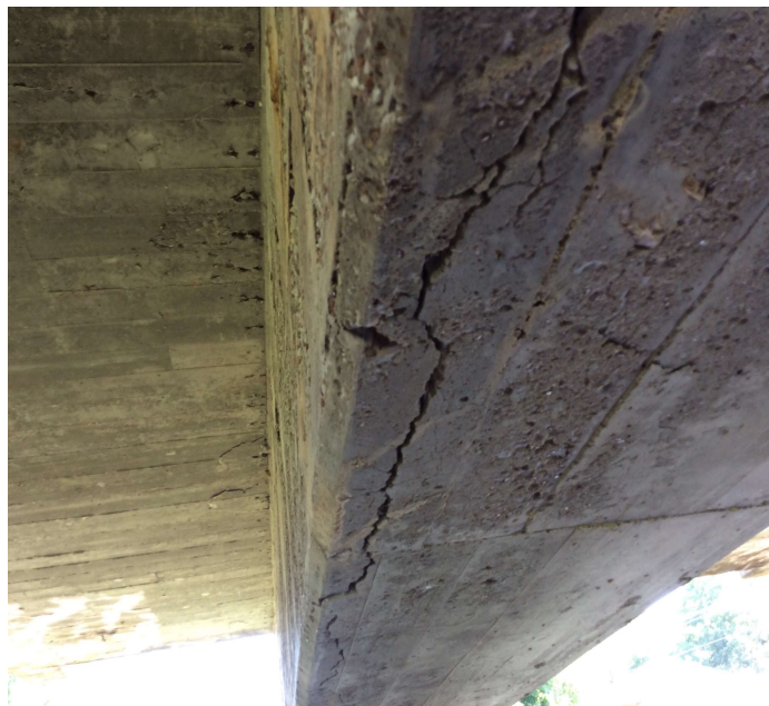
PHOTO 1 Description Large delaminated area to bottom of cap @ Bent 1.
