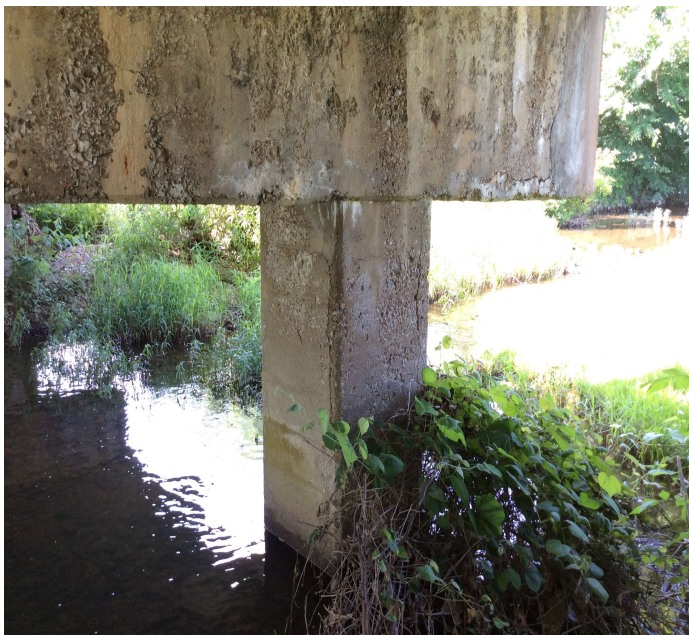
PHOTO 1 Description Vertical cracks to Right column @ Bent 1.
