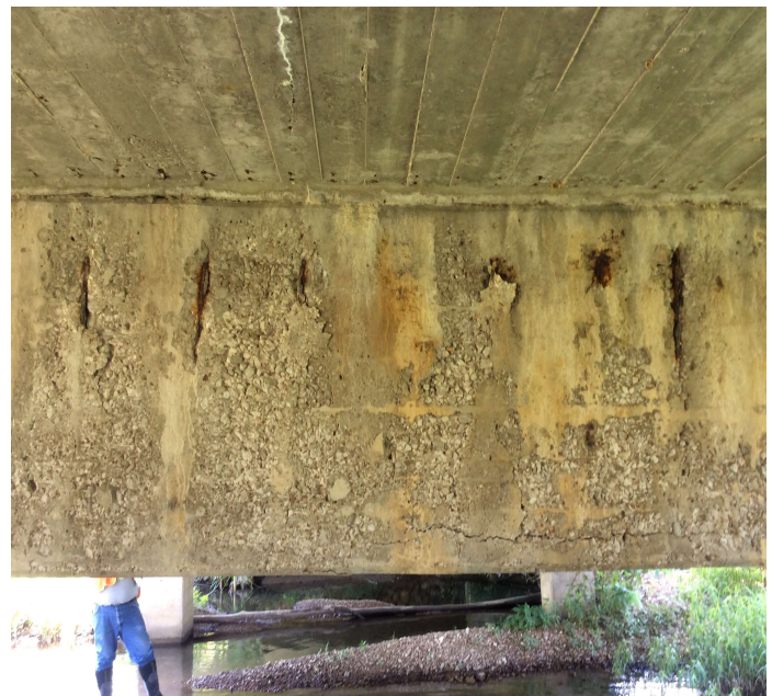
PHOTO 2 Description Exposed rebar to backside of cap @ Bent 1.(section loss is present)
