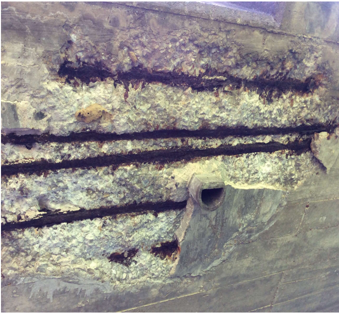
PHOTO 1 Description Spalls with rebar exposed to soffit @ Right side of Span 1.
