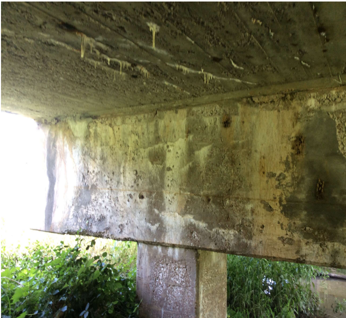
PHOTO 4 Description Efflorescent cracking to ahead side of Cap @ Bent 3.
